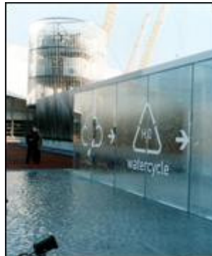
The dome water recycling system
